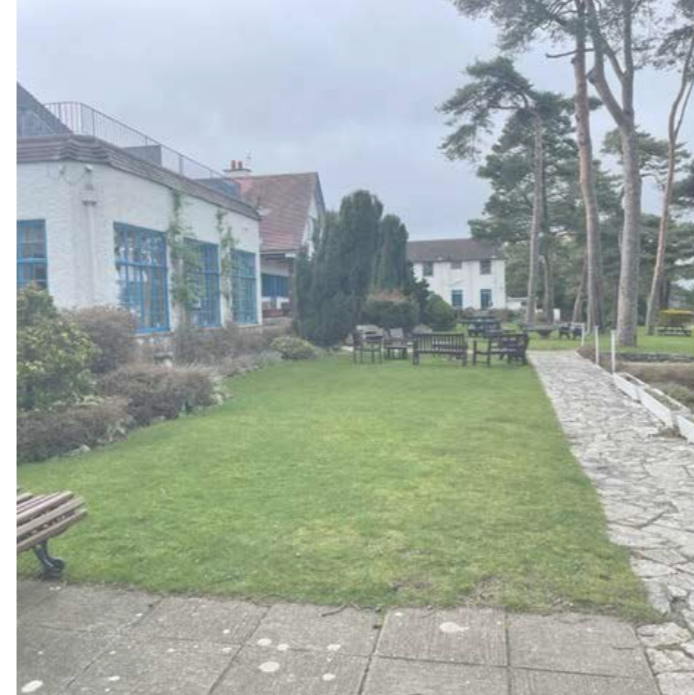
3. Existing garden terrace
