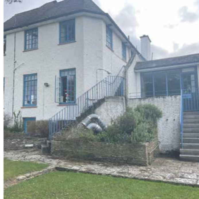
2. North of existing hotel facade
