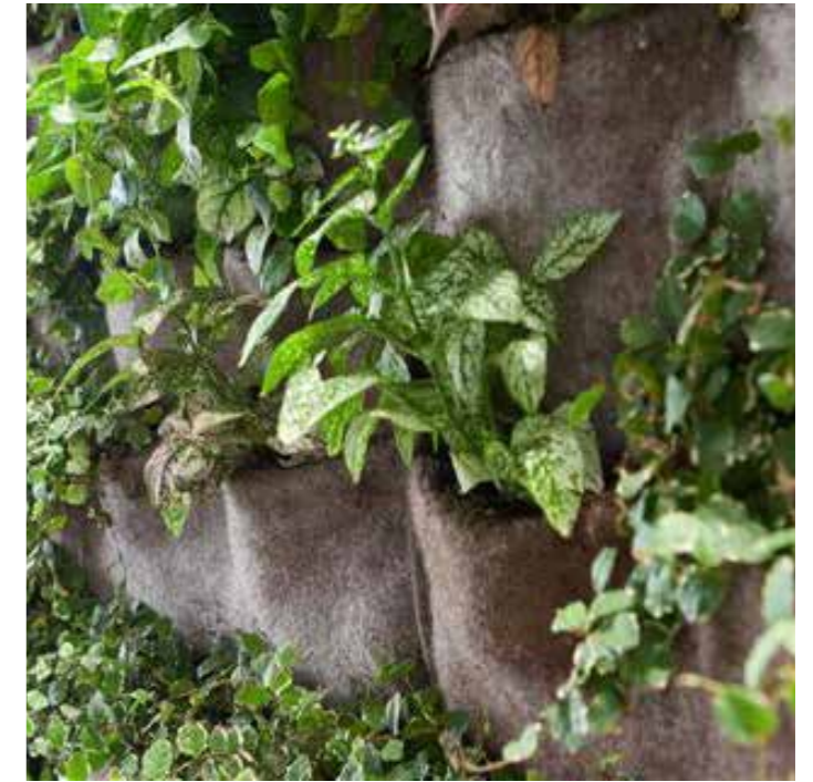
West planted retaining wall
