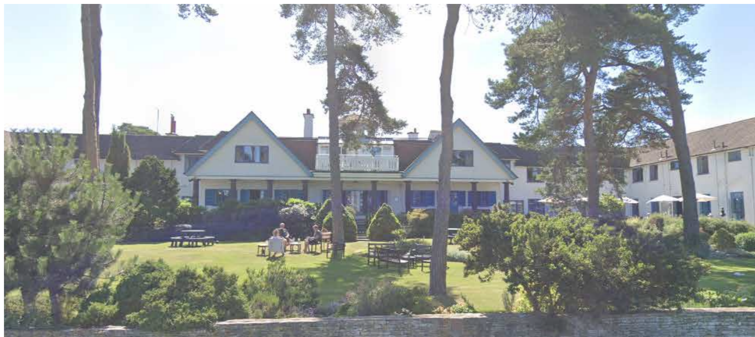
Elevation fronting Ferry Road
