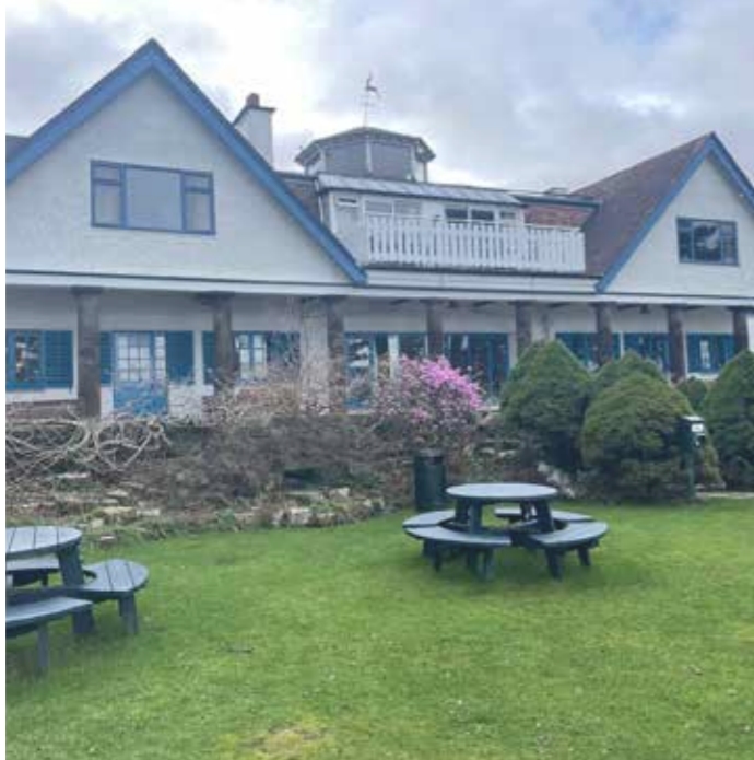
1. Existing east facade of hotel building
